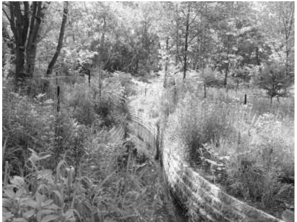
Gabler’s Creek flowing through the re-routed culvert at Aurora Pond. (The Douglaston & Little Neck Historical Society)
