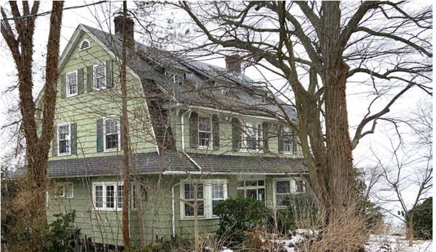
A gambrel-roofed Dutch Colonial at 15 Shore Road was designed by the architect George H. Hardway. The Japanese katsura tree in the front garden is one of the oldest in New York.
