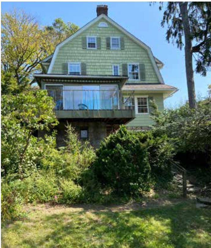
From the west side, the house is a full four stories including the attic.
