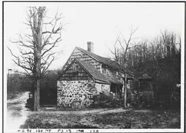
Foster House, near Alley Pond, December 7, 1900
